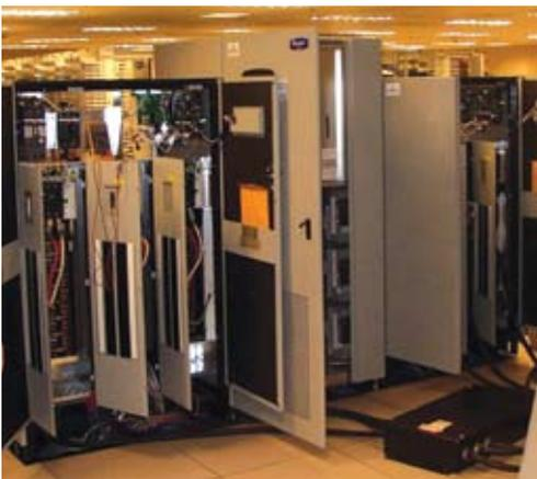
Figure 5 - Data center power distribution unit (PDU).
