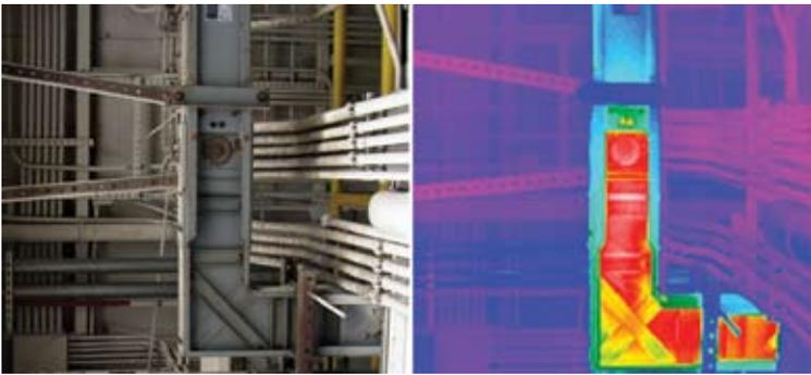
Figure 4 - Main buss duct with major heating problems.
